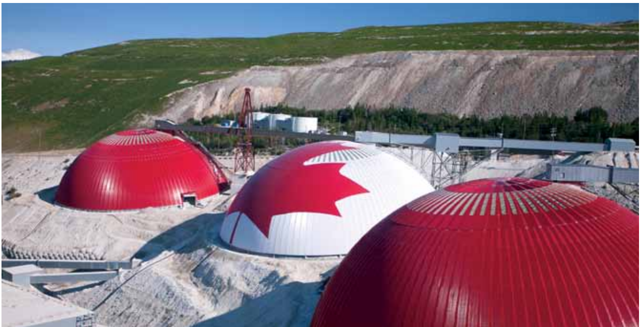
Pictured above: domes at Highland Valley Copper Operations cover ore stockpiles
