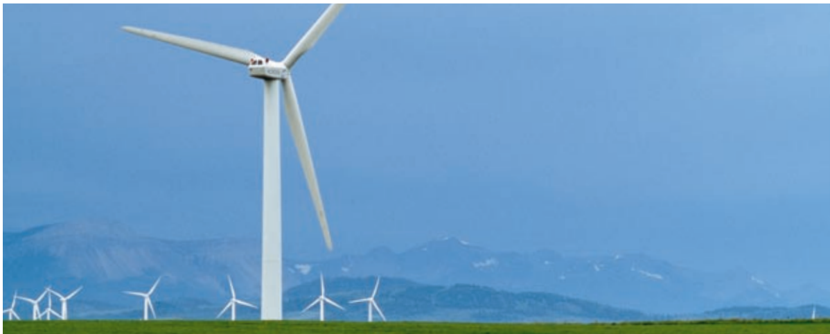
Wind Turbine Generators, Castle River Wind Farm in Cowley, Alberta. More than 170 tonnes of hard coking coal is needed to produce the steel in the tower which supports the blades as they generate electricity.
