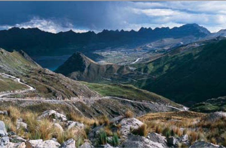
Overview of tailings pond and complex
