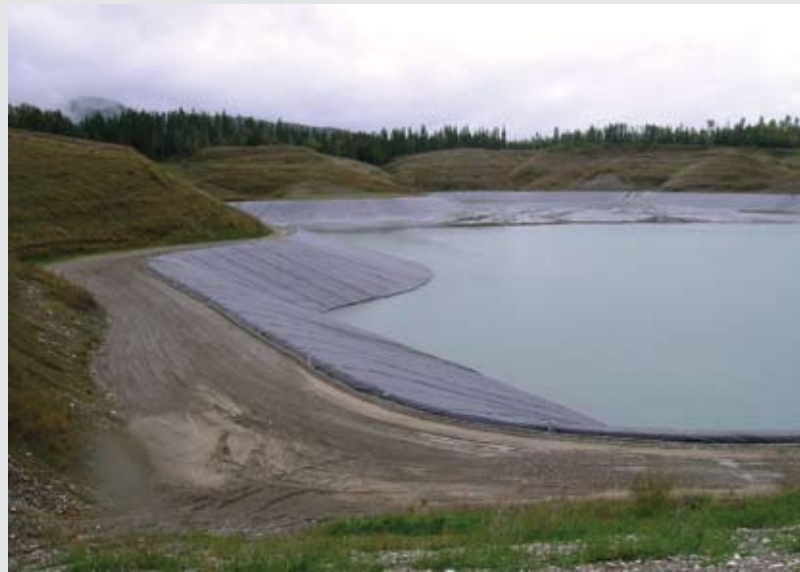
Double-lined tailings pond at Pend Oreille mine
