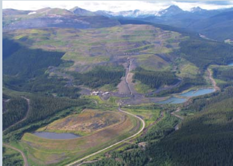
Reclamation efforts continue at the former Bullmoose mine
