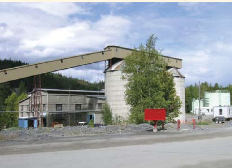
Pend Oreille mine surface facilities
